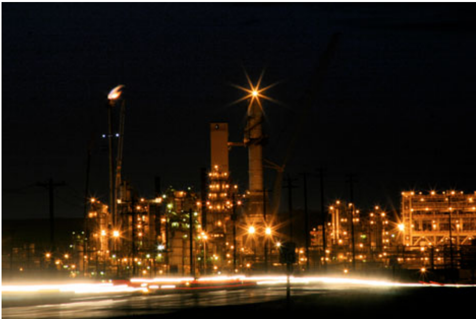
A Syncrude oil sands extraction plant in Alberta. (The Pembina Institute / David Dodge)
